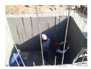
Our NGO chairperson and construction supervisor have been working with the local villagers to get the 15,000 litre underground water tank concreted and plastered. This work was completed in mid- May.
