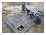
The tank is finished, the roof on and the inspection hatch since sealed. The piping is laid to the toilet block: and the pump is rigged up and ready. This tank will enable the school to capture and utilise the spring water, which feeds it all year round. When we are able we are planning to extend the supply to the kitchen and hostel.
